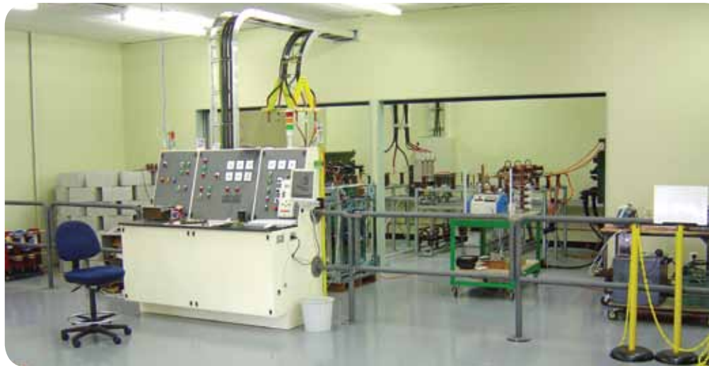
AuCom's medium voltage testing facility
